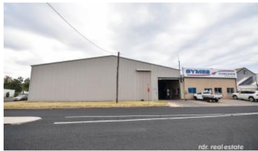
37 Mansfield Street, Inverell
