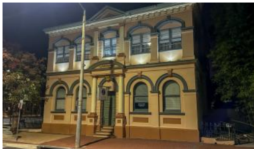
83 Otho Street, Inverell
