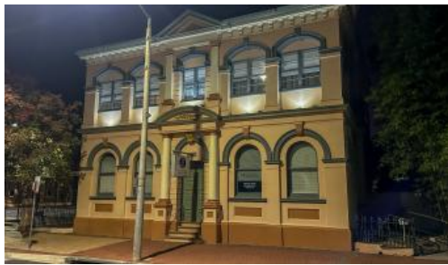
83 Otho Street, Inverell
